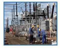
Regular sampling and testing of insulation oil taken from transformers is a valuable technique in a preventative maintenance program. If a proactive approach is adopted based on the condition of the transformer oil, the life of the transformer can be extended.
