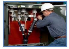
Cable terminations and joints form the weakest link in any distribution system. Also, a failed joint in an underground distribution system is much more difficult to locate and repair compared to any similar problem in overhead distribution systems. This means that we should do our utmost to achieve a good joint or termination, which can give years of trouble-free service.
