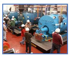
Power boilers, which are high-pressure boilers are mostly for power generation, industrial process and other applications where steam or high-temperature water is required. A power boiler is defined as a boiler in which steam or other vapor in generated at a pressure of more than 15 psi for use external to itself. Other power boilers include heat recovery steam generator, organic fluid vaporizer, electric boiler, miniature boiler and high-temperature water boiler.
